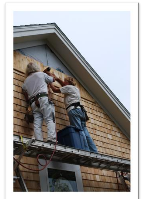
Sue and neighbor, Pilly, are at the very peak of the chapel as they nail the cedar shingles to the exterior wall.
