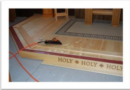
Floorboards and trim are added to the platform and the front is faced with the words “Holy, Holy, Holy”. Simple and beautiful at the same time.
