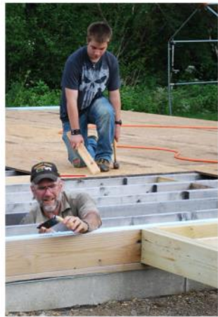
Fr. Alan and neighbor, Spencer, work on joists and subflooring.
