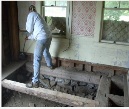
Mother Sue sweeping up 200-year old floor timbers during renovations.
